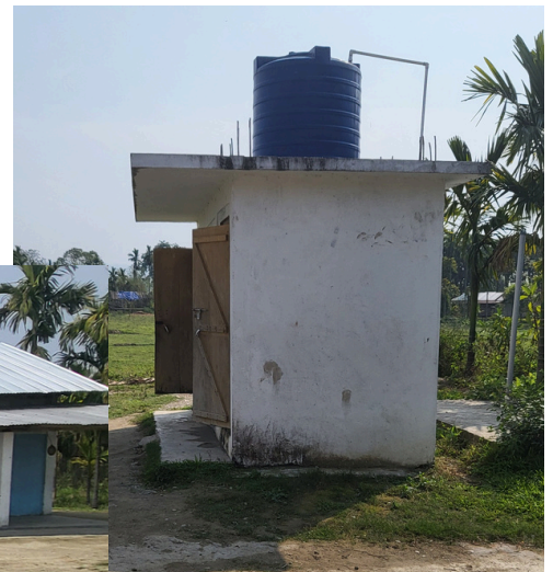
Toilets and Water Tank
