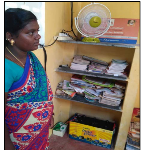
Solar PV system installed at single teacher school
